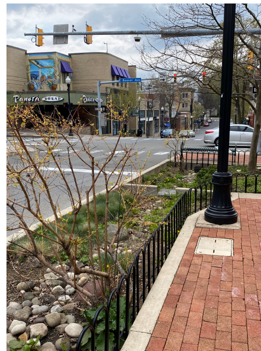
Fig. 12: Curbside rain garden in State College slows stormwater and acts as groundwater recharge
