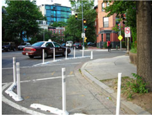
Fig. 4: Temporary plastic bollards, temporary curbs, and paint demark an expanded sidewalk: DDOT Completes Temporary Bulb-Outs: Greater Greater Washington
