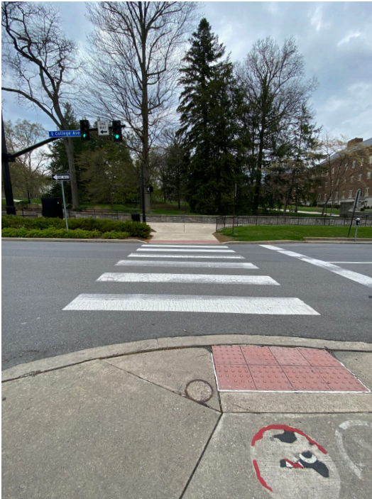
Fig. 6: Zebra stripe crosswalks in State College have higher visibility for pedestrians and drivers than outlined or unmarked crosswalks.
